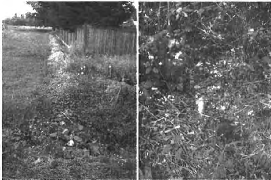
Large curtain drain (left) just uphill from the subject property. One of several drainage outfalls depositing onto the subject property from neighboring development (right). While difficult to see, a 4" PVC drain pipe deposits onto a pile of quarry spalls, located next to wetland flag A1.
