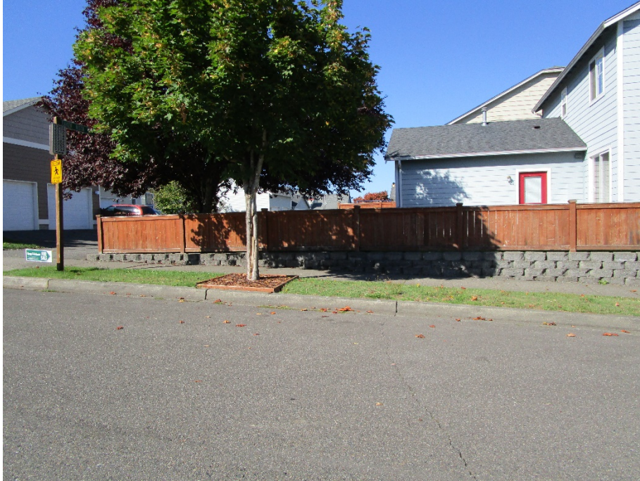
Small retaining wall with 42 inch fence on top – 33 rd St NE
