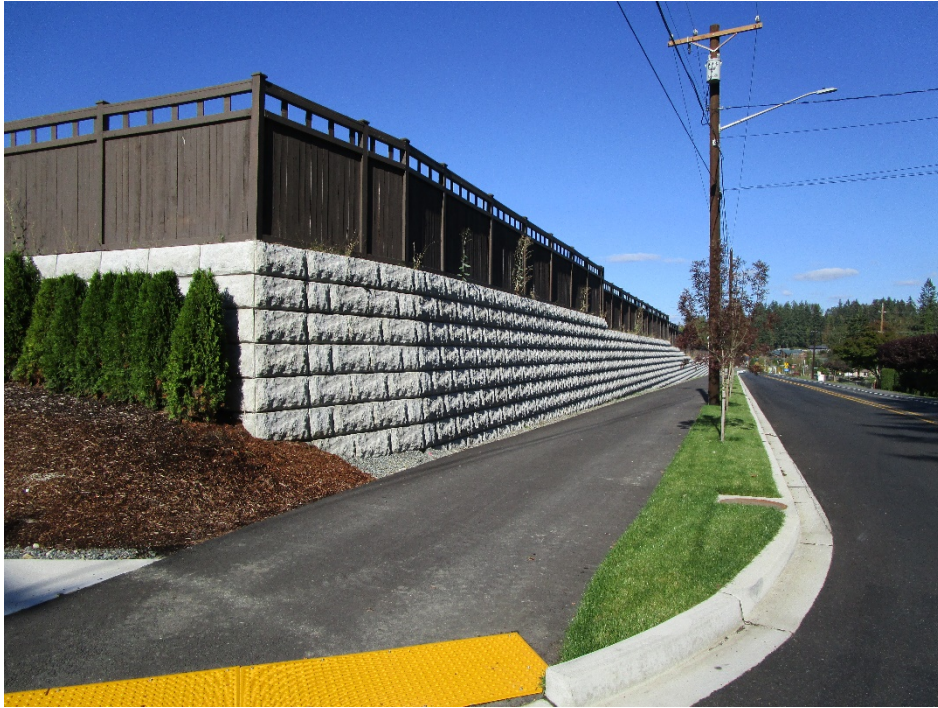
Fence/Retaining Wall Combinations - Daysala Plat – S. Lake Stevens Road and internal lots
