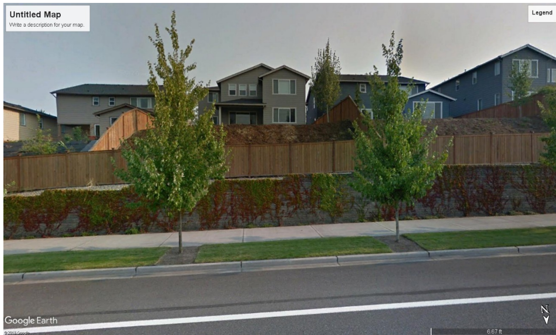
Retaining wall with gap behind then solid wood fence, grading to natural contours - Woodinville
