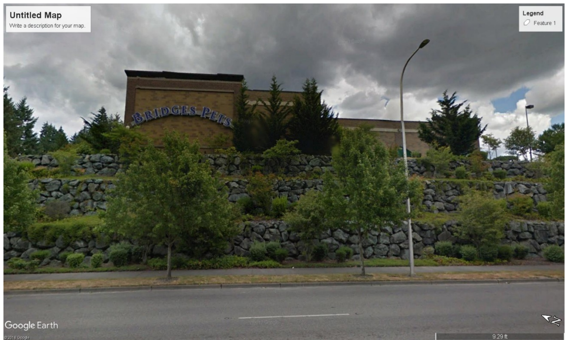
Terraced retaining wall with vegetation – Snohomish Station
