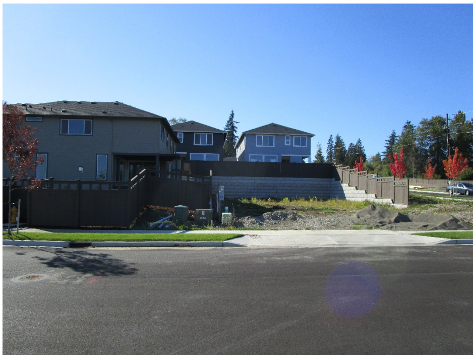
Fence/Retaining Wall Combinations - Daysala Plat – S. Lake Stevens Road and internal lots
