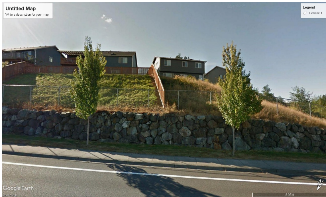
Retaining wall with chain link fence combo, grading to natural contours – Ingraham Blvd, Marysville
