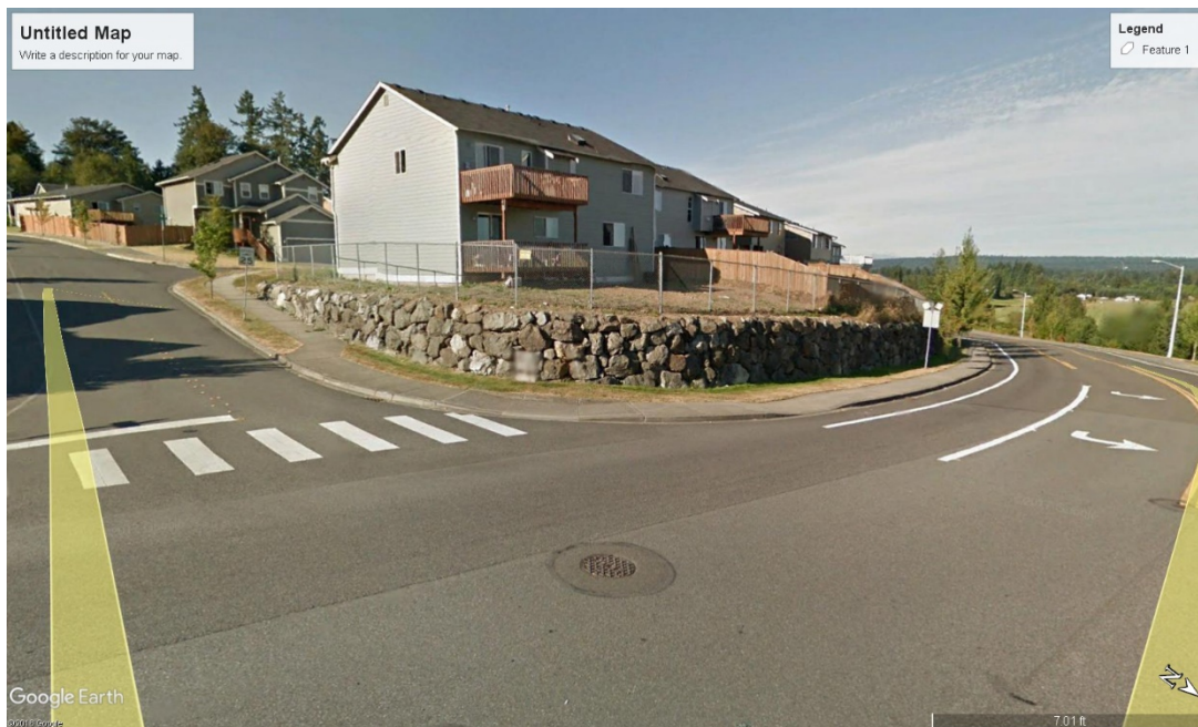
Retaining Wall/Chain-link Fence Combination – Ingraham Blvd, Marysville
