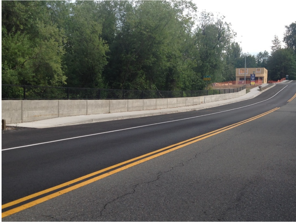
Retaining Wall/Chain-link Fence Combination – 99 th Ave SE
