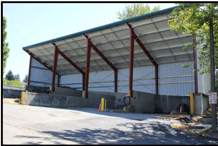
Kirkland decant facility designed by PACE Engineers
