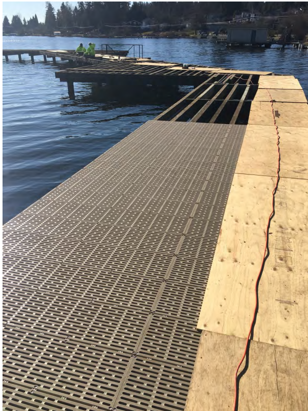
Dock restoration underway
