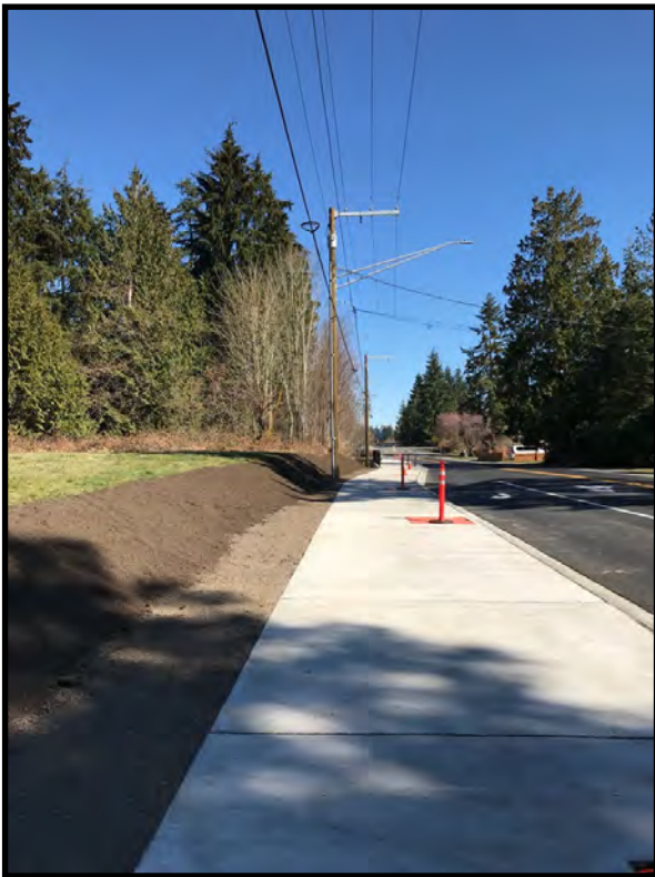
91st & 4th safe route nearing completion March 2019
