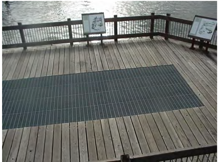
Figure 6: The City of Raymond's community pier includes grating to allow light to reach the water. Photo by Barbara Nightingale.
