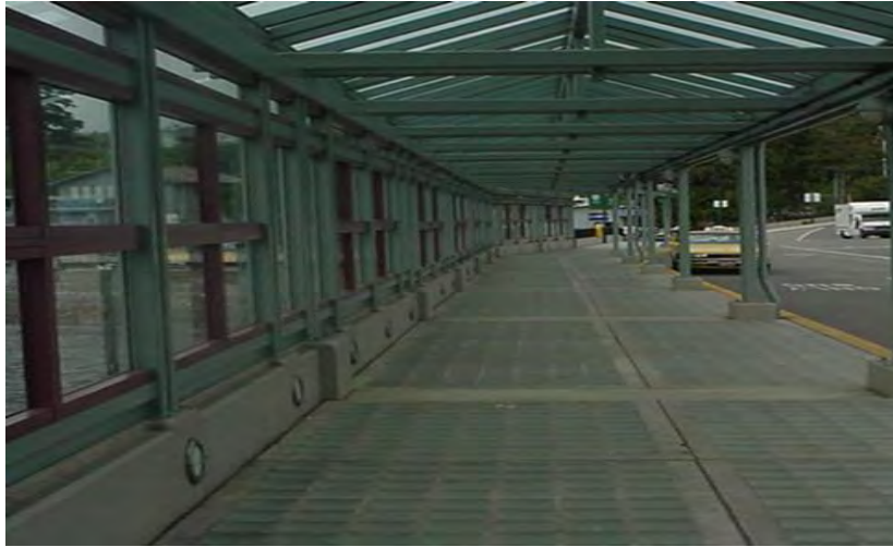
Figure 5: Glass blocks at the Clinton ferry terminal allow light to pass through to the water below. Glass blocks must be kept clean to be effective. Photo by Barbara Nightingale.
