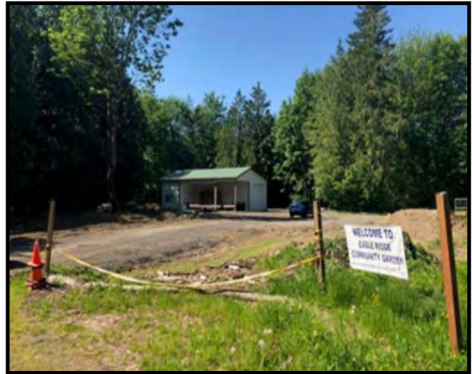
Eagle Ridge Park Parking Area—May 2018
